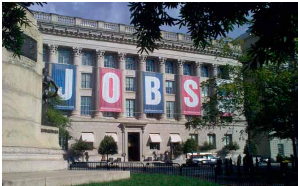
US Chamber headquarters at H and 16th Streets.
